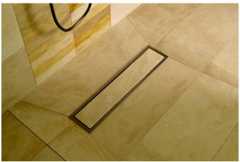
Linear drain—cover filled with tile.
